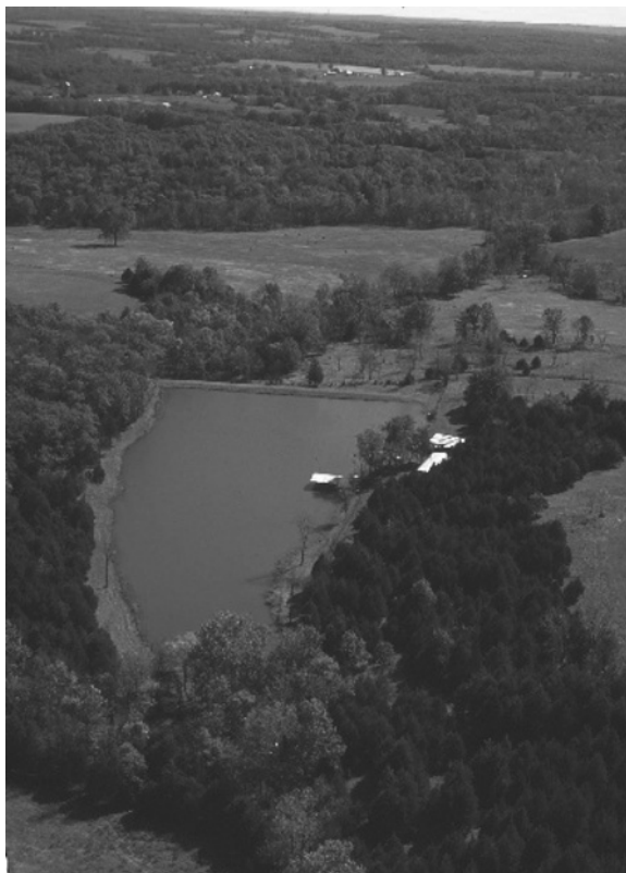
Figure 1.2 A watershed lake in Western Missouri provides water supply (Courtesy of the National Resources Conservation Service and USDA).
